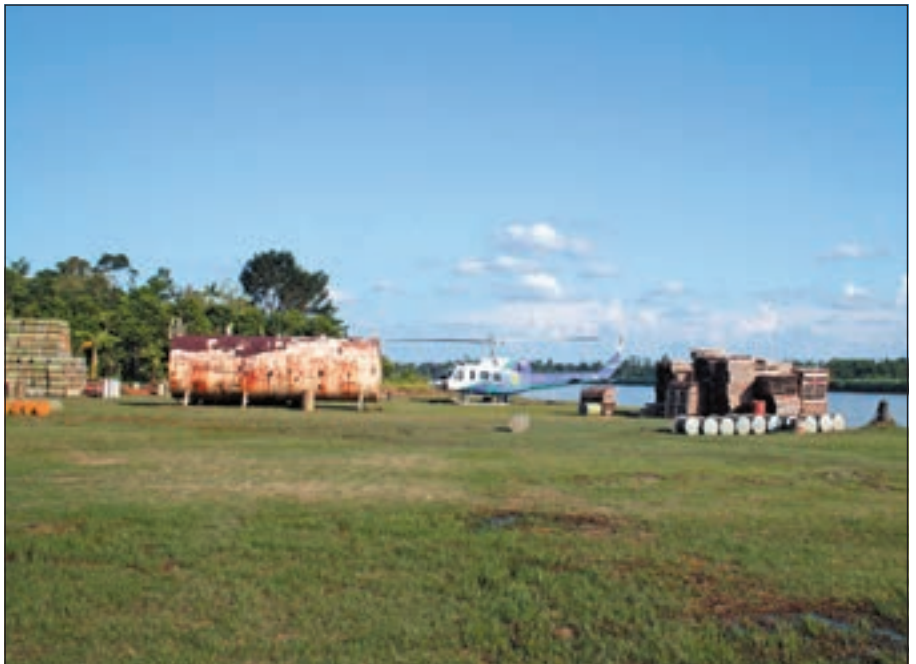
Plate 46 Barge loading and fuel storage facilities at Iniook
