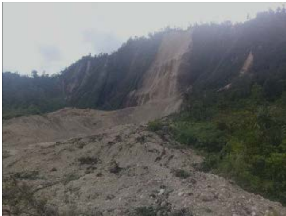
Figure 3-103: Failure in the epicentral area triggered by 25 February 2018 earthquake
