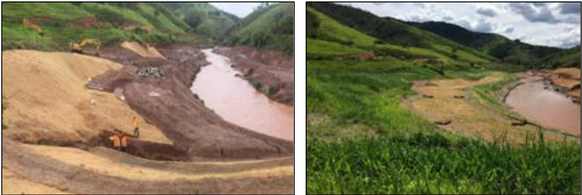
Figure 14-2: Bio-engineering of erosion-prone slopes (photos taken in Minas Gerais, Brazil)
