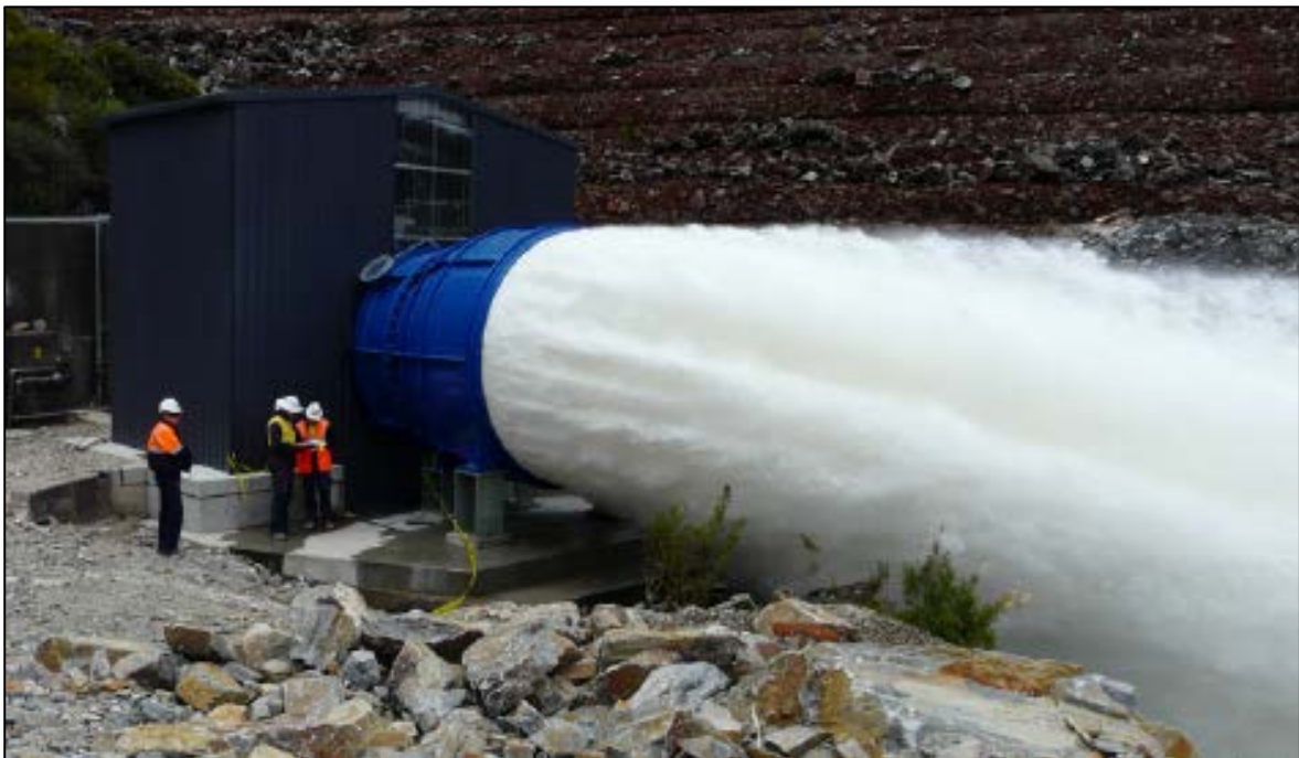
Figure 16-11: Fixed cone dispersion valve
