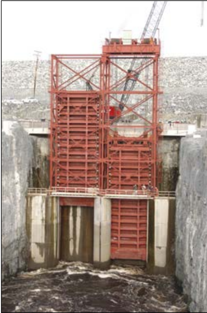
Figure 10-9: Wheeled gate diversion structure 85
