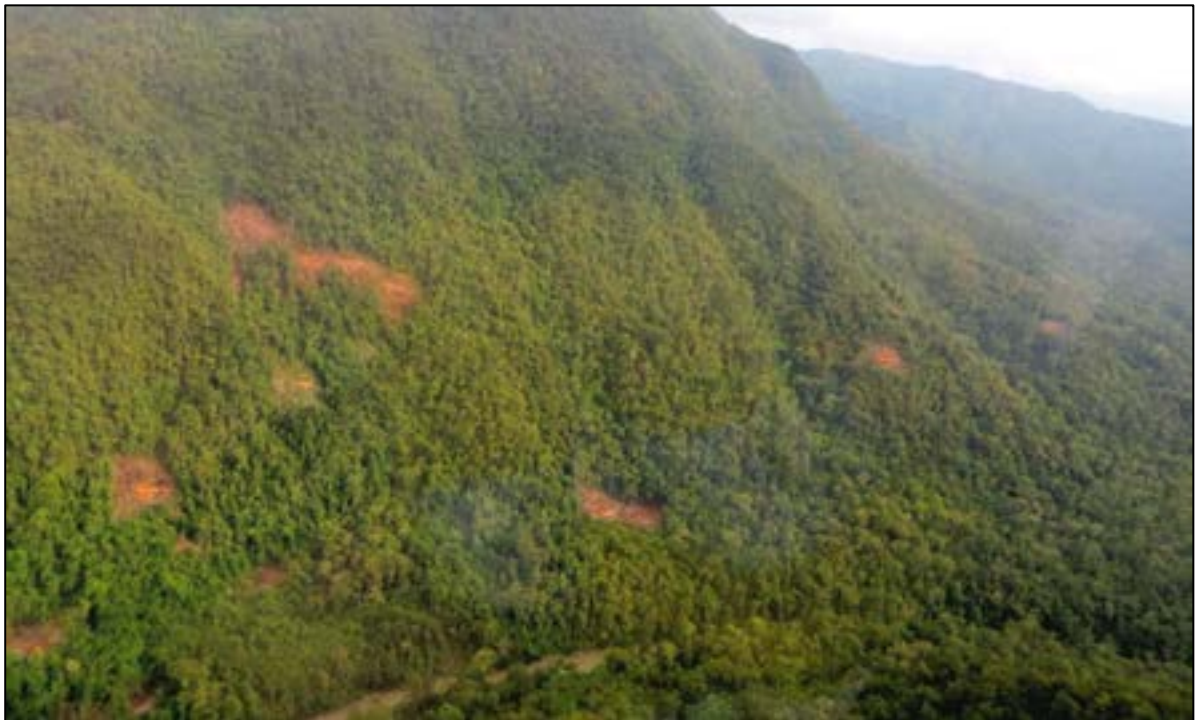
Figure 3-18: Photograph of the steep right abutment, looking southeast, showing drill pads
